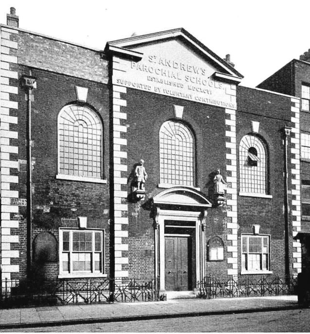
School buildings—1696. In use as a church school until the war. Bombed in February 1944
